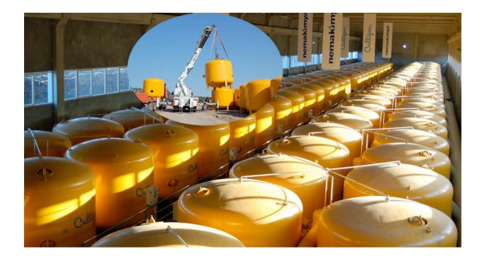
A recently completed, extensive water filtration project in Izmir, Turkey was installed by Nema Kimya, a member of Turkey's Nema Holding group of companies. This project utilizes 12,500 cu. ft. of GreensandPlus<sup>™</sup> from Inversand Company, Clayton, NJ USA as the filter media in the arsenic removal process.
